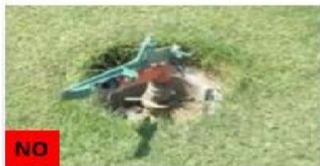
Exposed irrigation head
