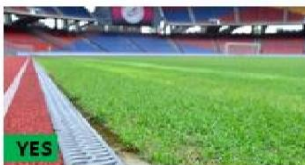
Proper drainage cover
